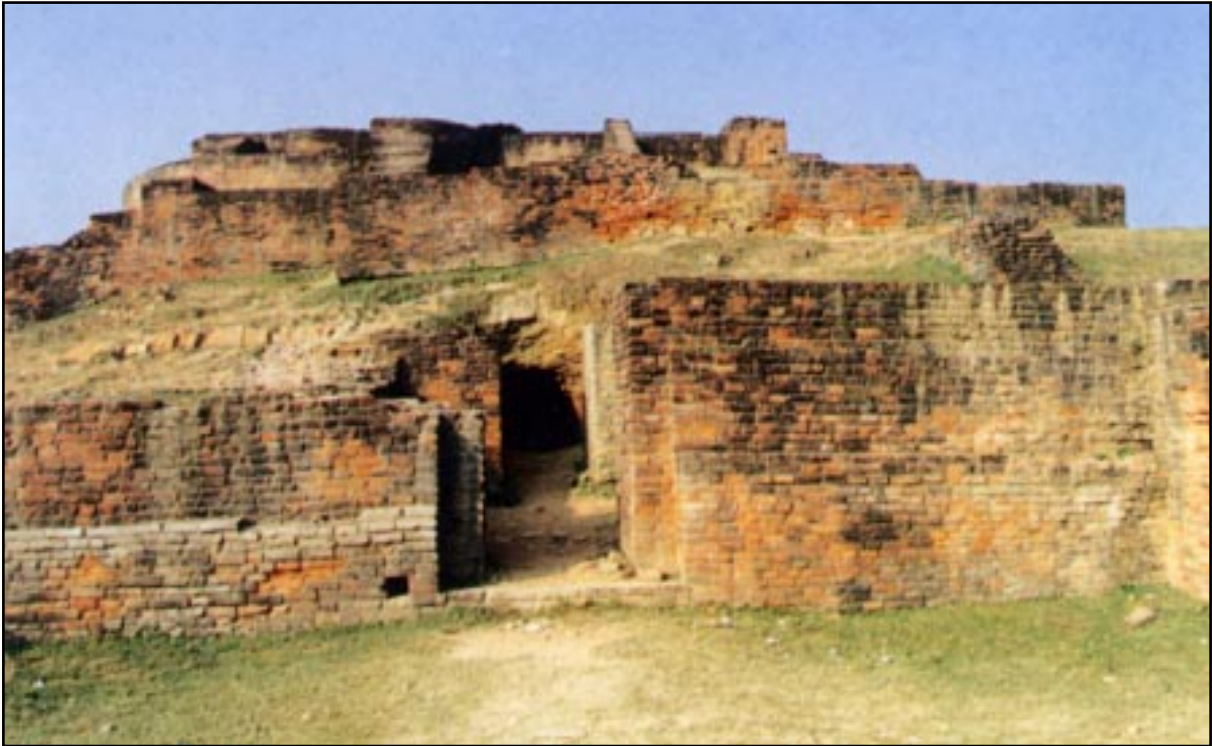
Plate 27. Sravasti. The Angulimala stupa at Mahet, showing the opening of a tunnel cut through its base for drainage. RETURN
